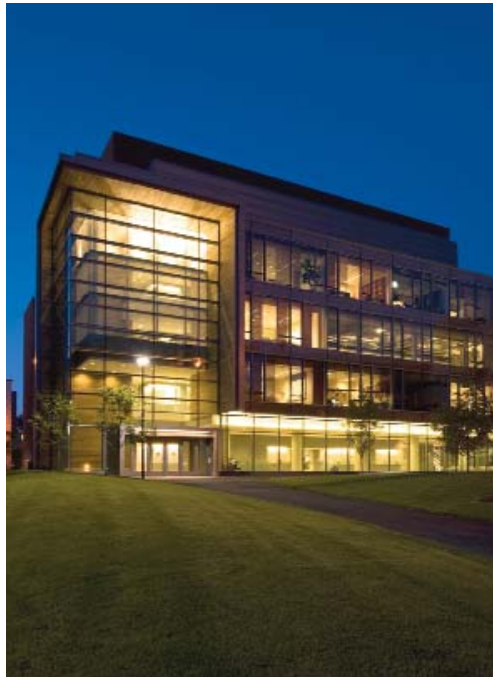
Harvard University Faculty of Arts & Sciences , 500,000 sf Northwest Science Center and Central Energy Plant. ( SOM )
